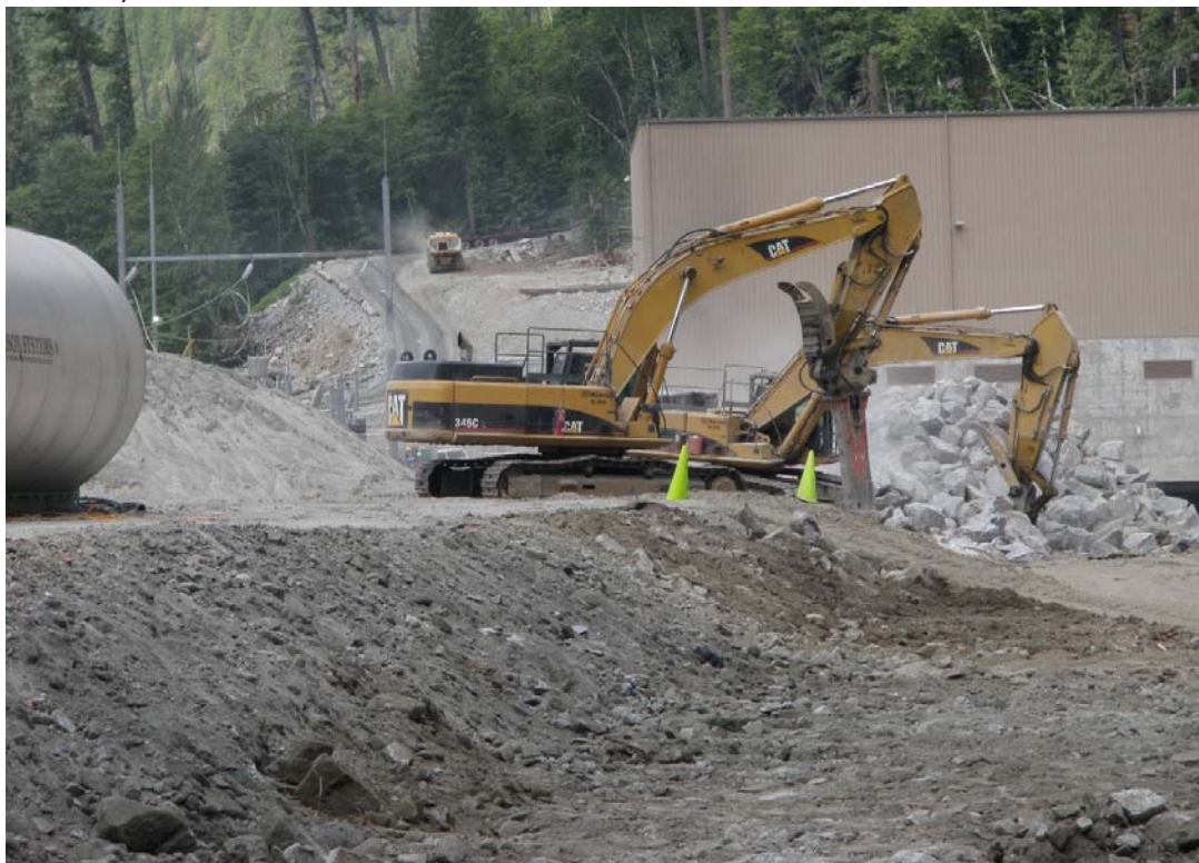
(Photo 2) Breaking and stock piling riprap at the Montrose powerhouse. (July 11, 2010 12:25)
